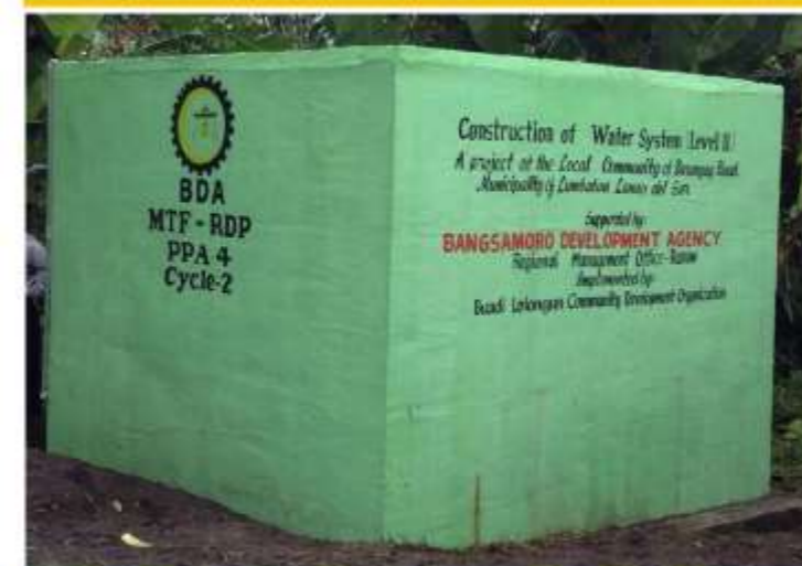
Water System (Level II) established in Brgy. Buad, Lumbatan, Lanao del Sur with 1,020 beneficiaries
